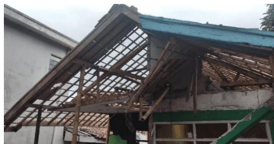
Figure 6: Failure of Connections in the Wooden Roof Frame
