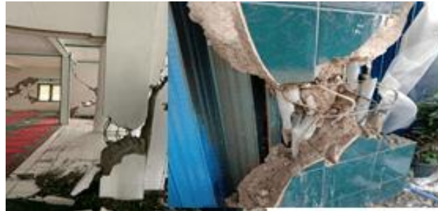
Figure 8: Failure in Rebar Hook Installation in Columns
