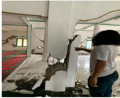
Figure 3: Column Structure Failure Unable to Support Beam and Roof Framework
