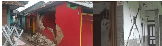
Figure 5: Photo of Wall Collapse Due to Poor Design and Lack of Anchors/ Reinforcement in the Columns to Bind the Wall
